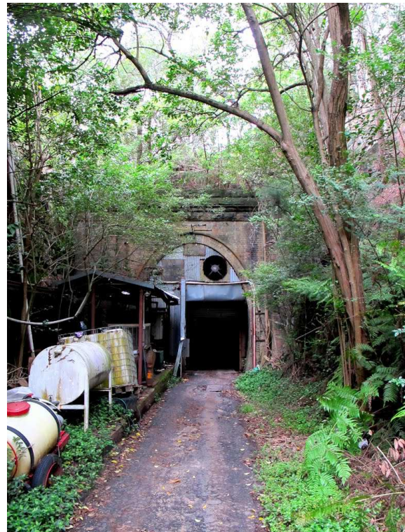
Glenbrook Old Railway Tunnel: Western Portal
