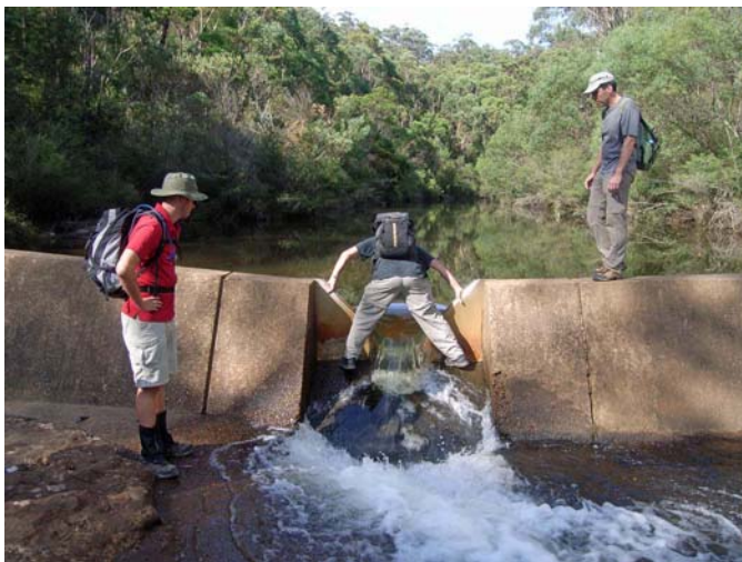
Straddling the spillway
