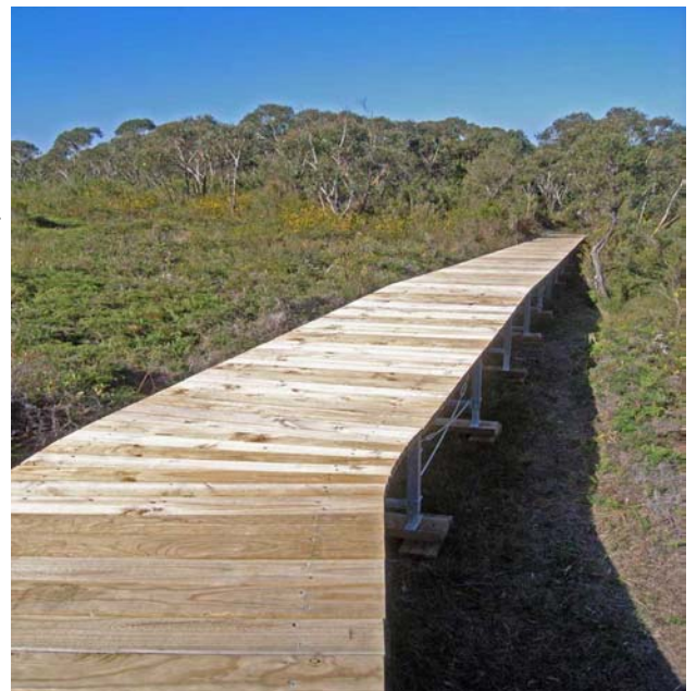
Newly constructed boardwalk
