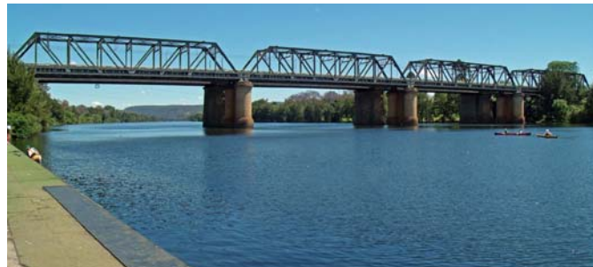
Victoria Bridge - NE side
