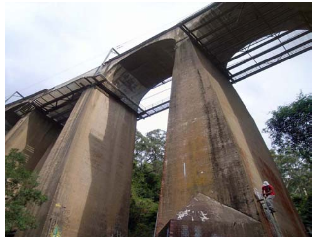
Stanwell creek Viaduct
