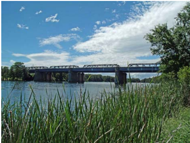
Victoria Bridge - SW side
