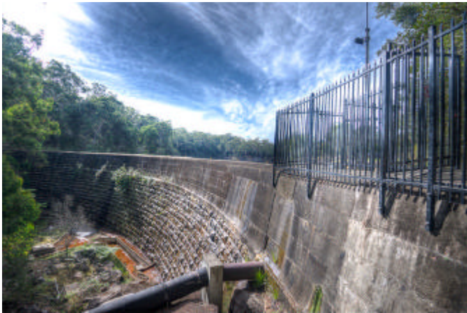
Masonry dam wall
