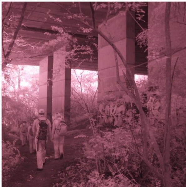
De Burghs Bridge Art Gallery
