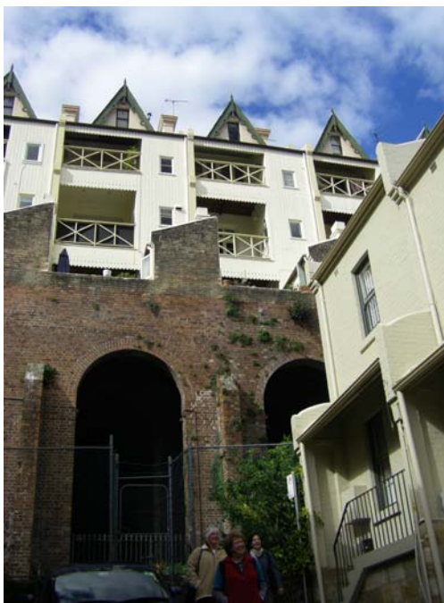
View from the back of the terrace houses in Victoria Street
