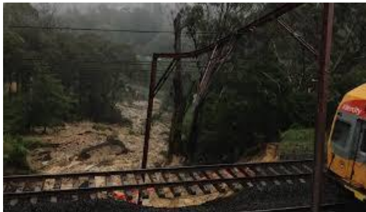
SLIP: The extent of the damage caused by a landslide on the track between Leura and Katoomba. Photo: PAUL TOOLE MP
